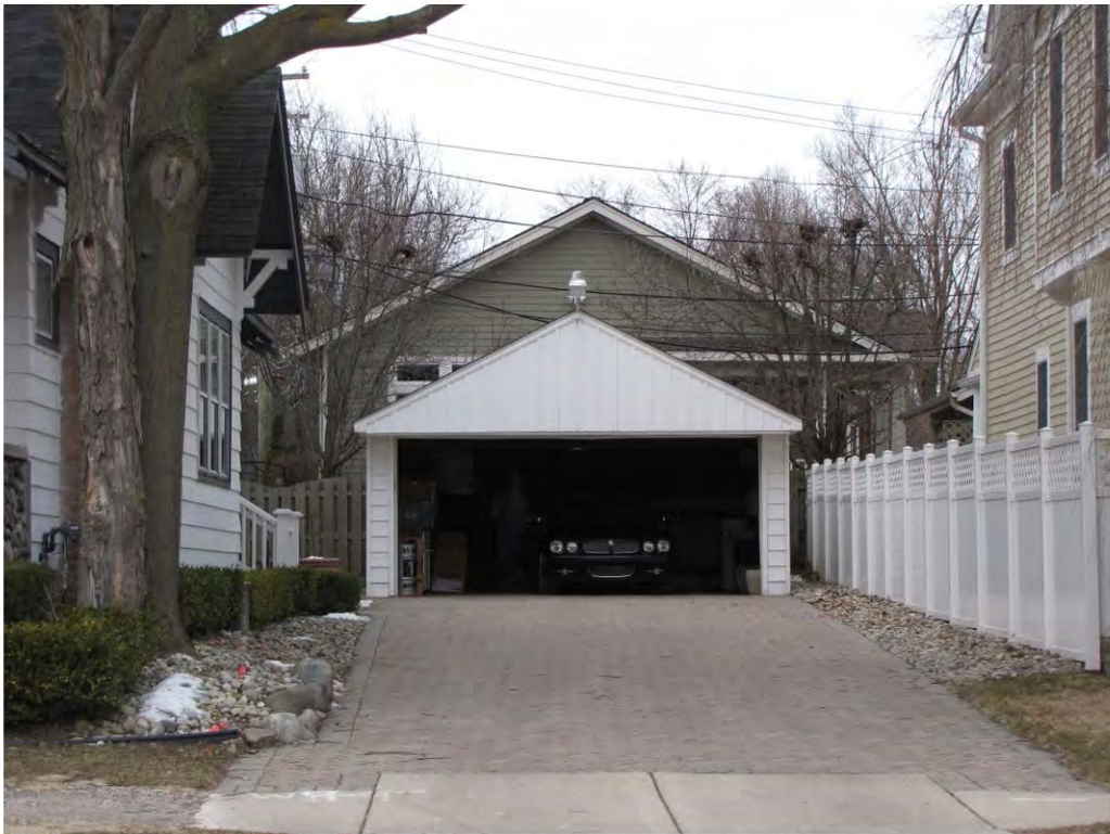
Wing North 111, Garage_Looking West
