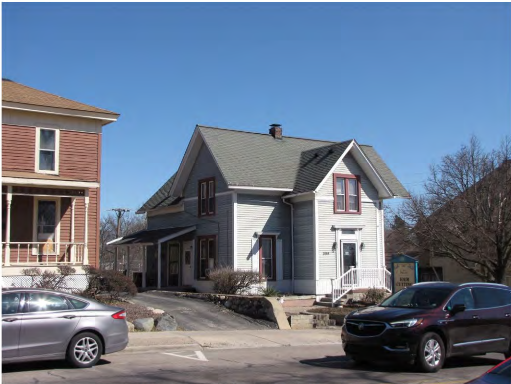
Main East 355_ Looking Northeast
