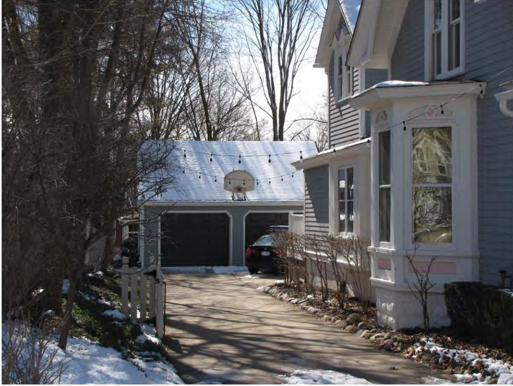
Main West 521, Garage_Looking South
