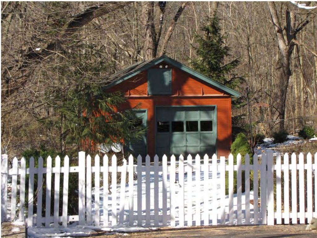
Rogers North 201,Garage_Looking West
