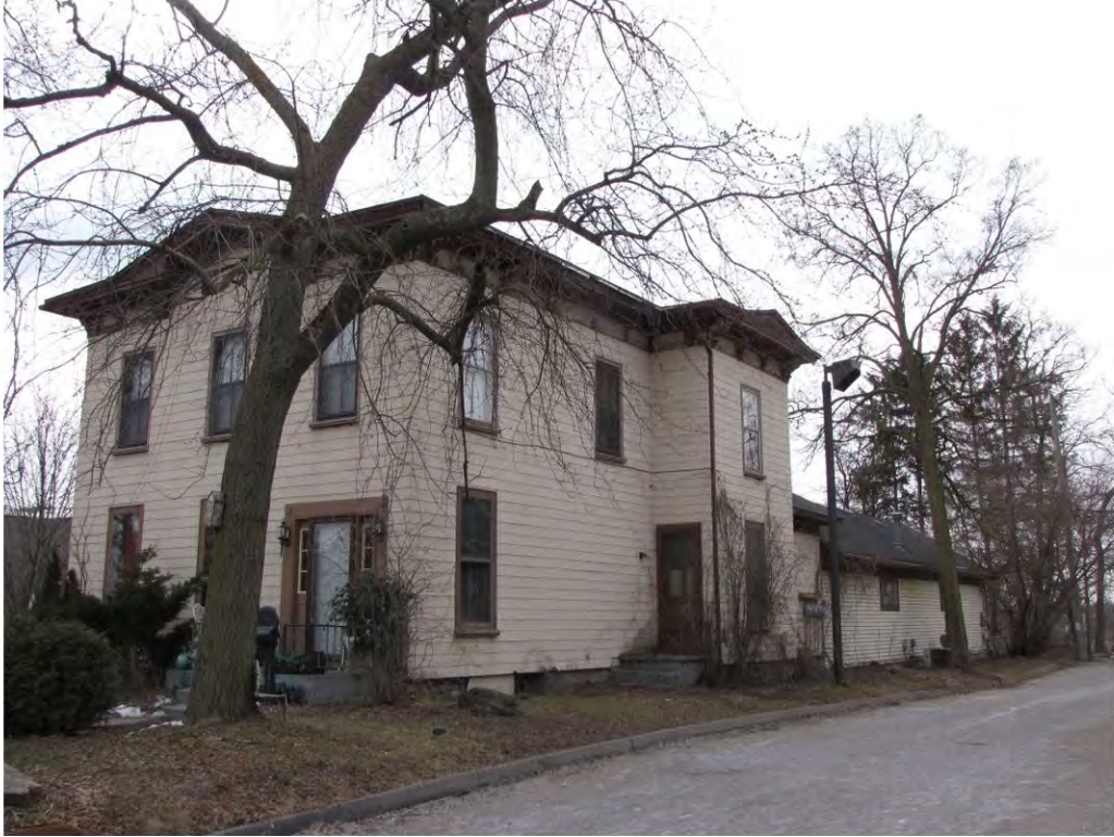
Main East 342_ Looking Southeast
