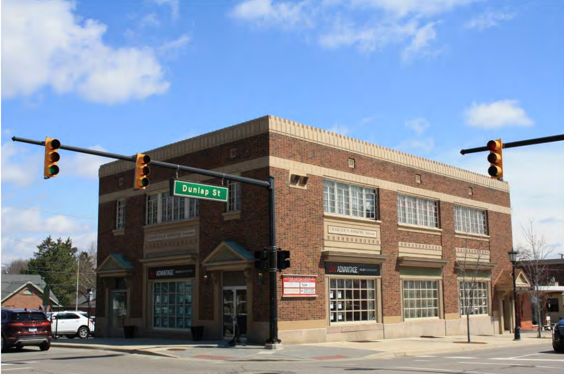
Center North 200_Looking Northeast
