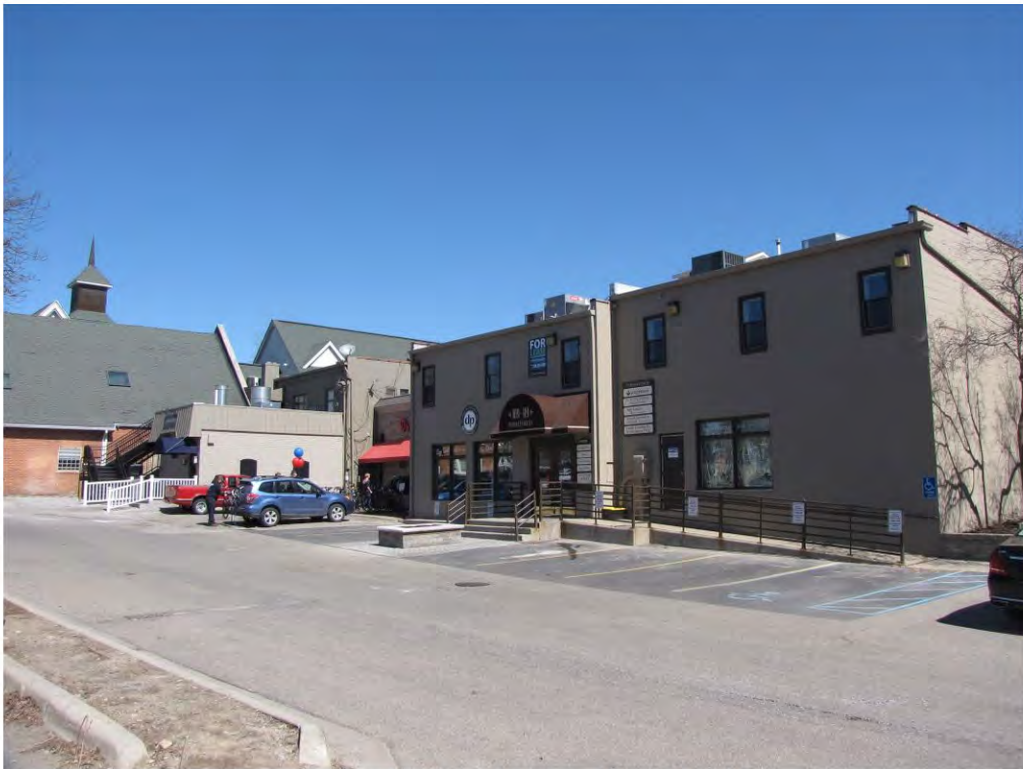
Center North 109-115_Looking Northeast
