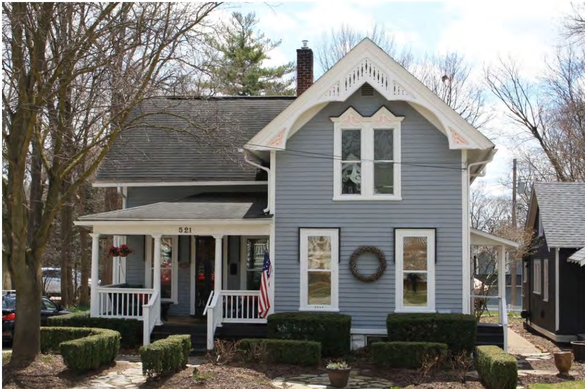
Main West 521_Looking South
