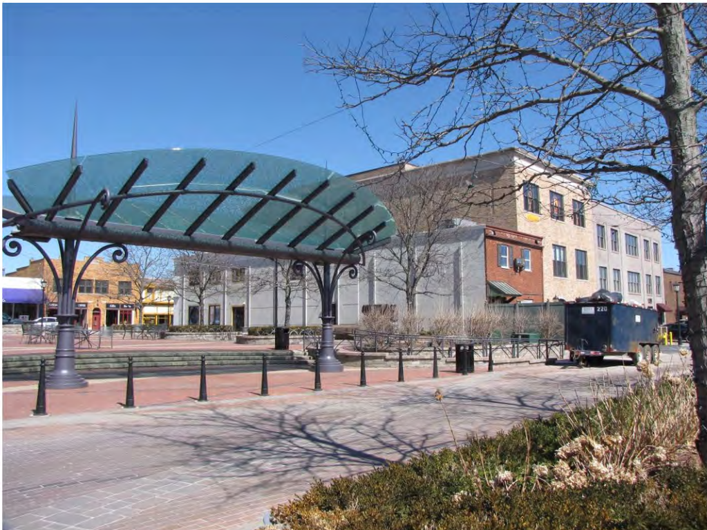
Main East 156 - 158_ Looking Northeast
