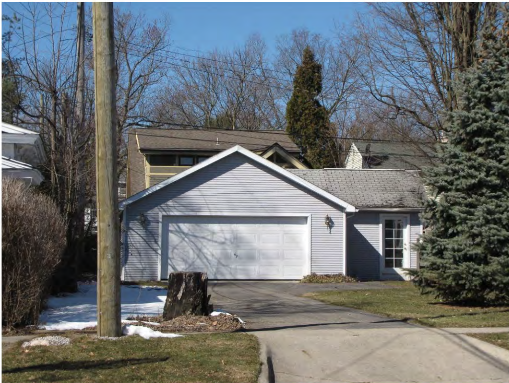
West 223, Garage_Looking West
