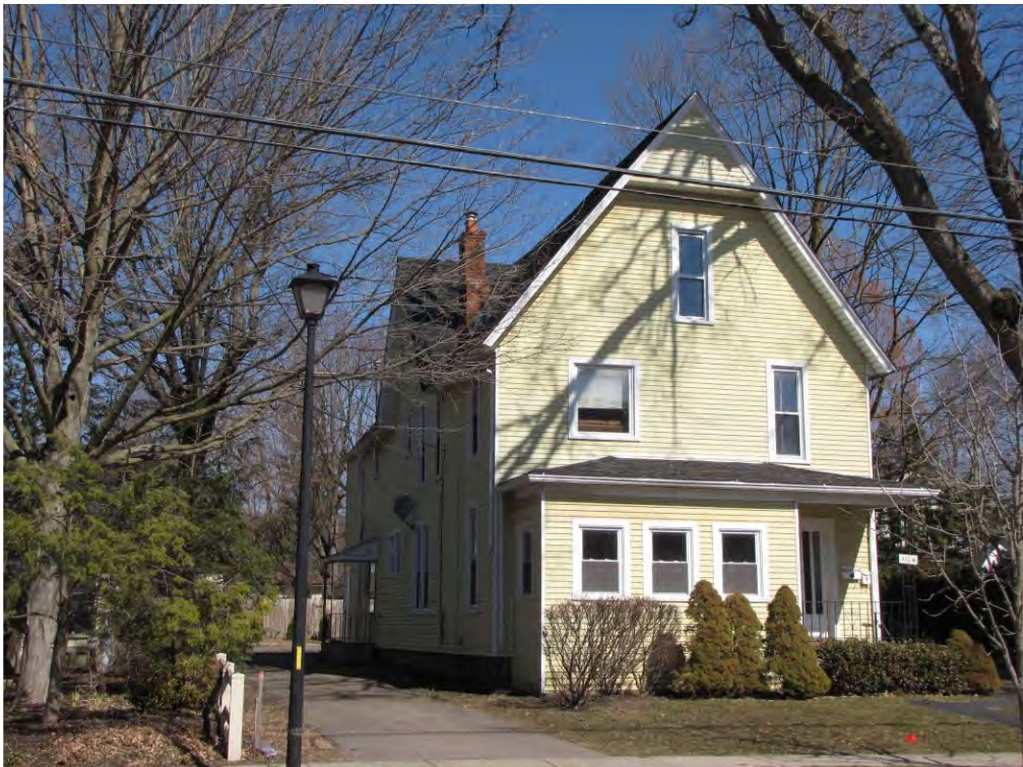
Main West 410_ Looking Northeast
