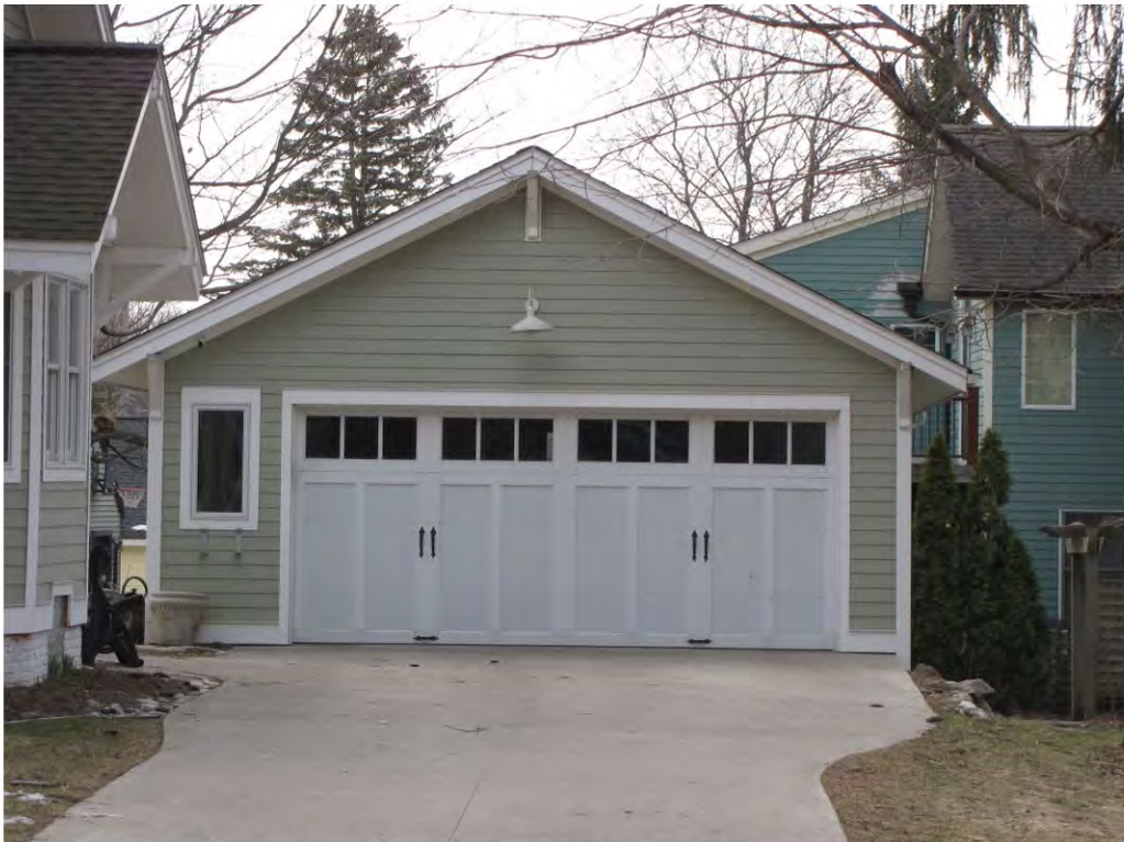
Cady West 487, Garage_Looking South
