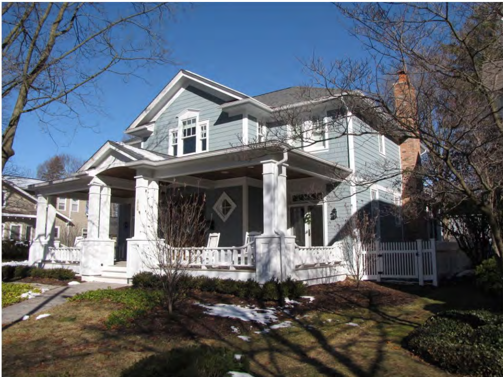
Cady West 500_ Looking Northwest
