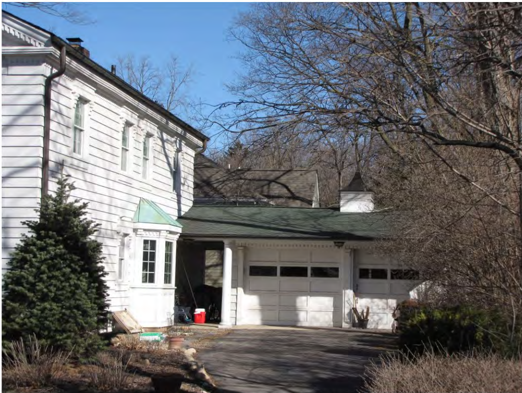
Randolph 204, Garage_Looking North
