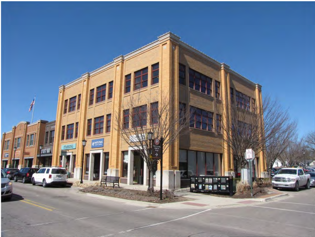
Main West 114-126_Looking Northwest
