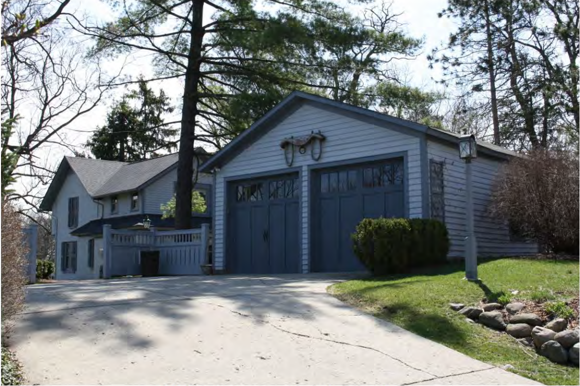
High 239, Garage_Looking Southeast
