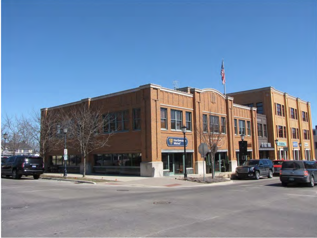
Main West 114-126_Looking Northeast
