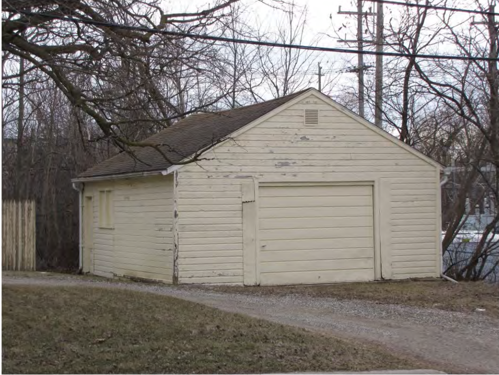
Cady East 350, Garage_Looking Southeast
