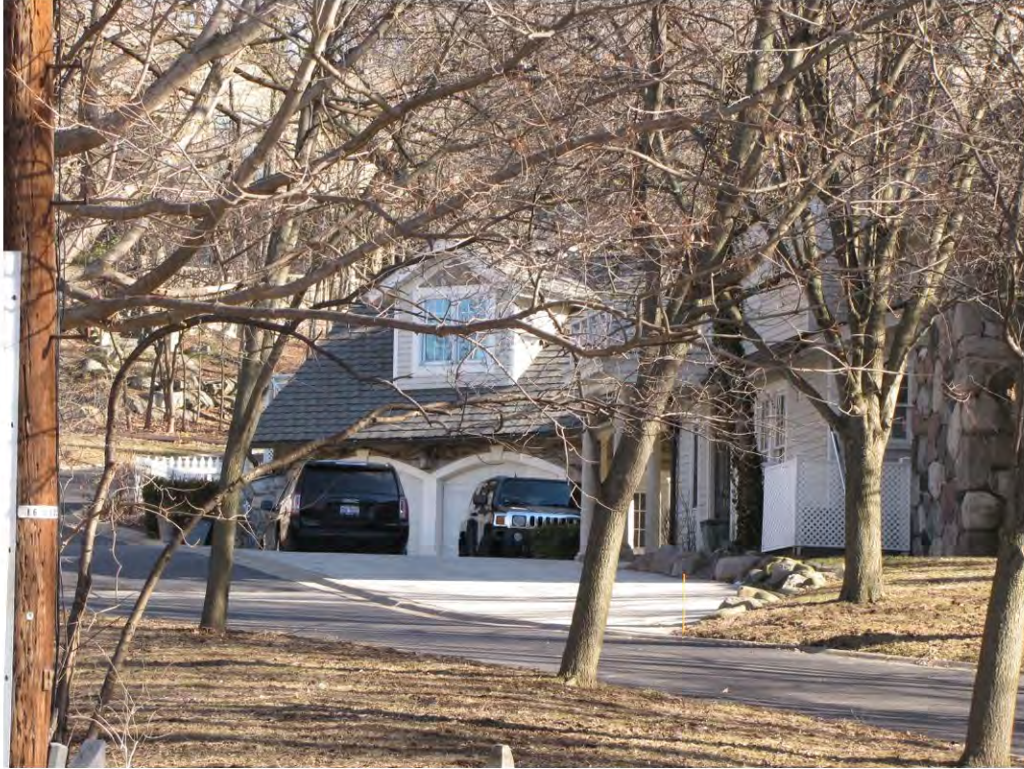
Randolph 562, Garage_Looking North
