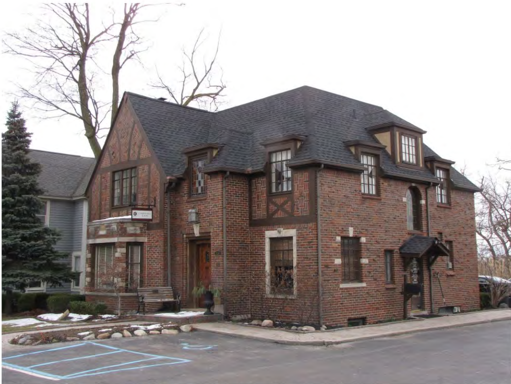
Main East 324_Looking Southeast
