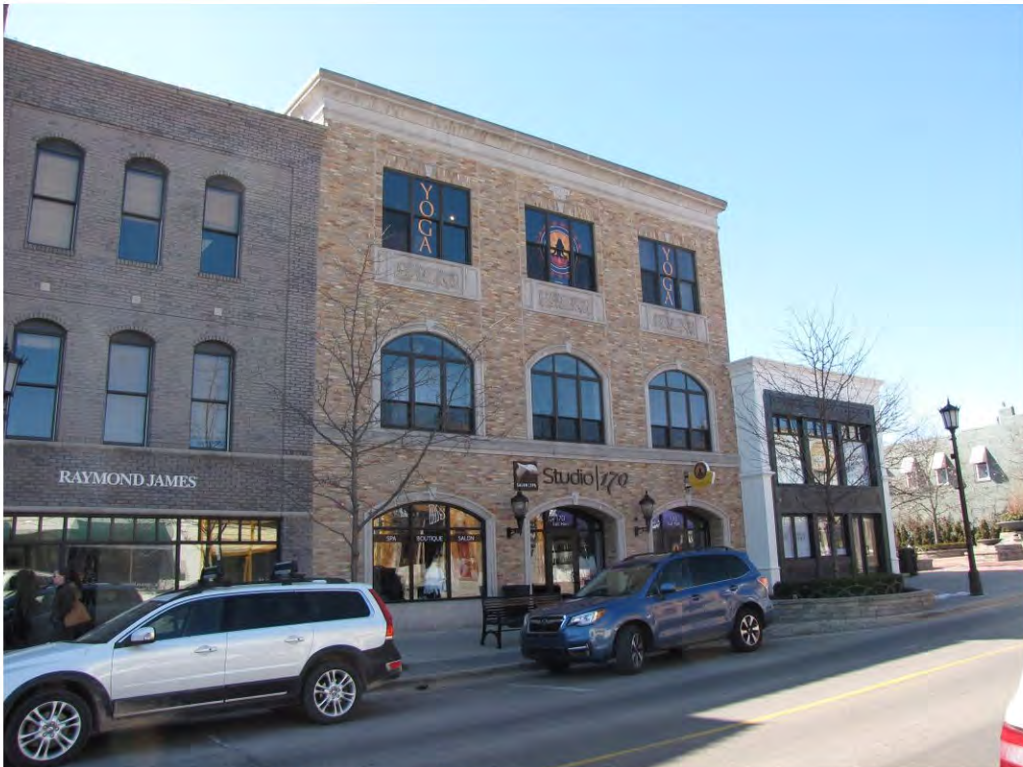
Main East 170_Looking Southwest
