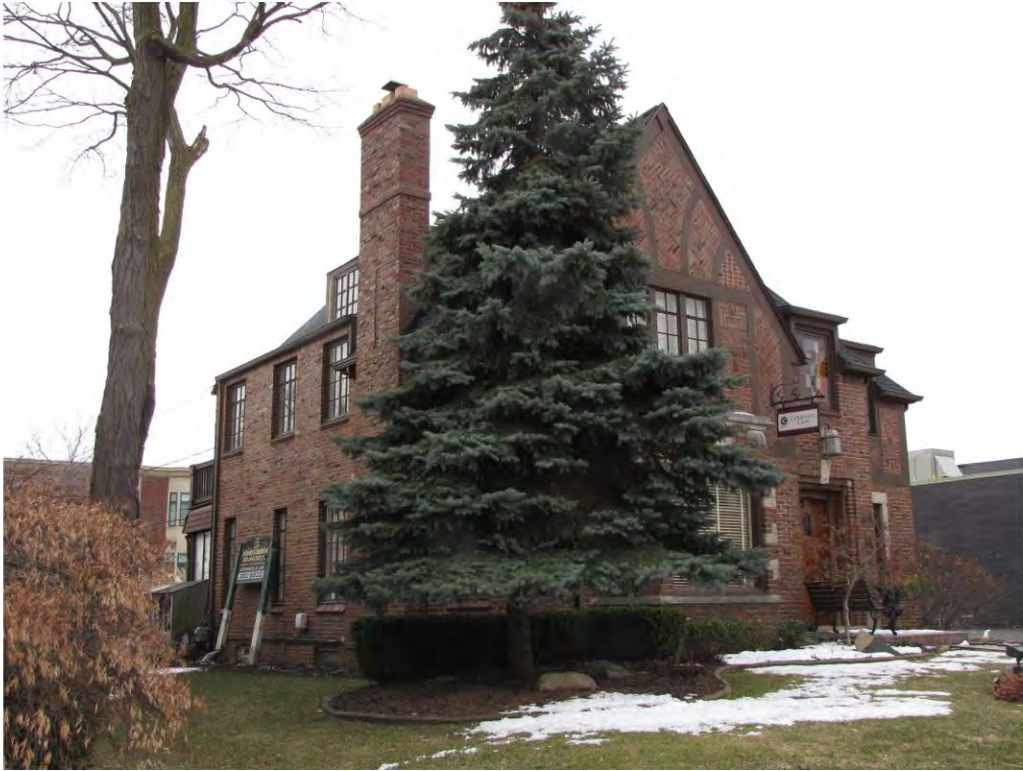
Main East 324_Looking Southwest
