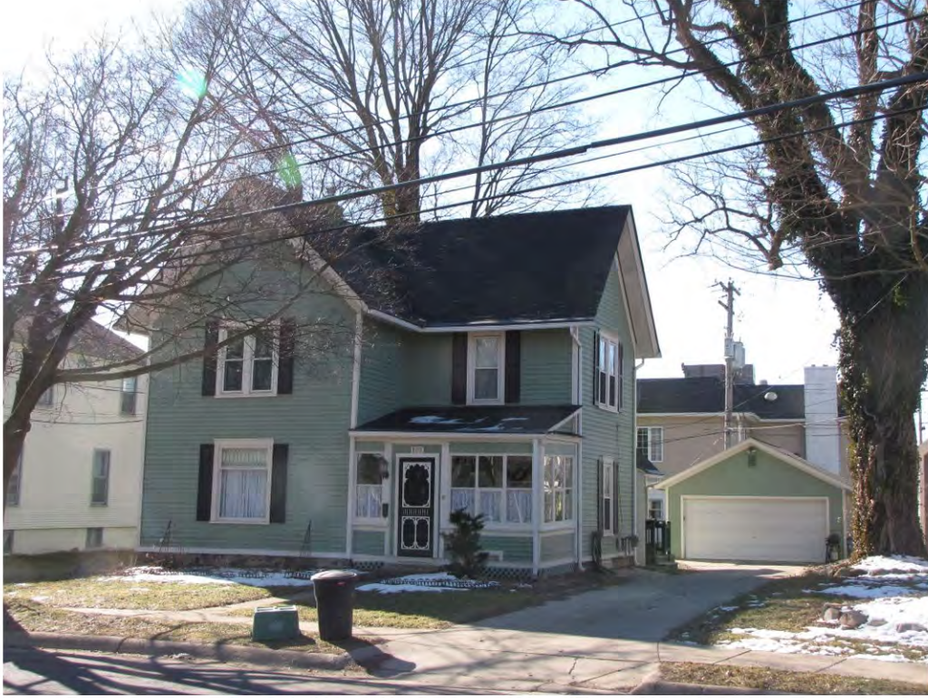
Randolph 125, Garage_Looking South
